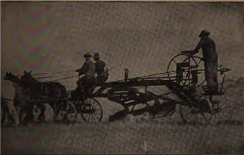
Reclamation Grader Commencing Irrigation Ditch. Figure 14.
